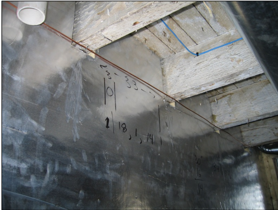
Figure 3. Foil-faced polyisocyanurate installed inside a basement wall
