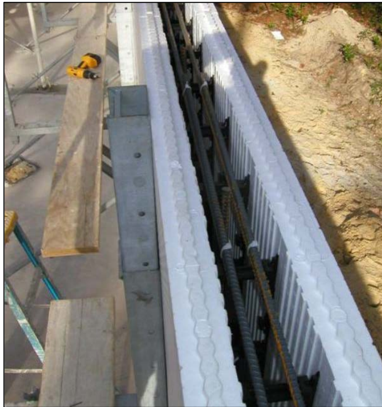
Figure 19. Insulated concrete forms before pour
