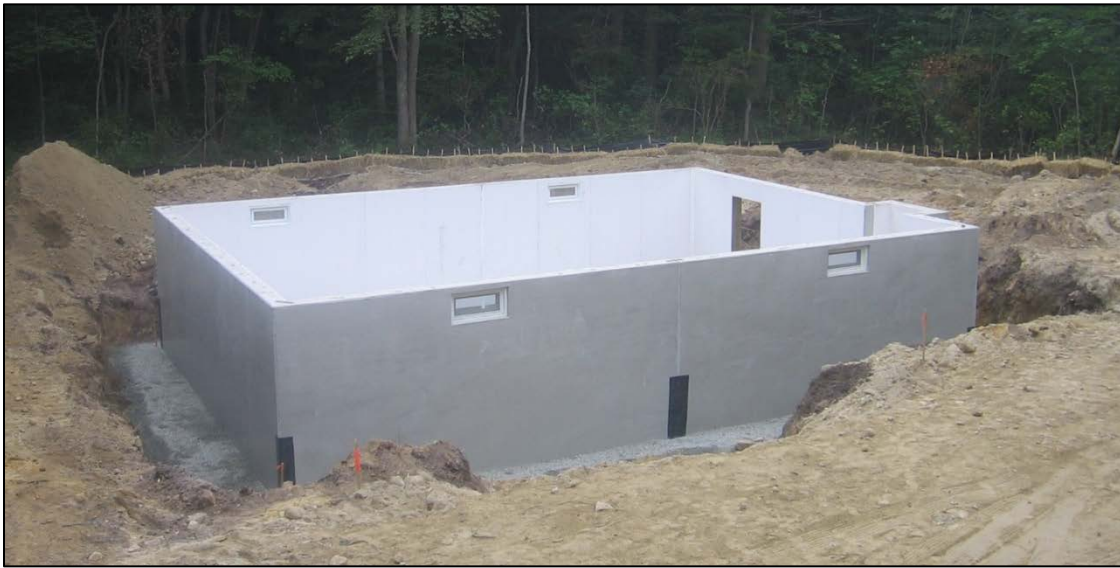
Figure 22. A completed, pre-cast, insulated foundation
