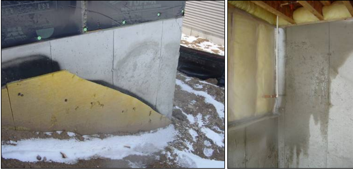
Figure 14. Exterior fiberglass insulation on this new home was cut to terminate below-grade after backfill. The inside of the wall showed significant condensation—and even ice—during cold winter conditions.
